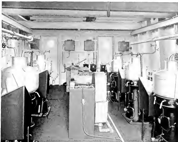
Seven De Laval oil purifiers for removing water from whale oil. Total capacity 35 tons or 6250 gallons per hour.
